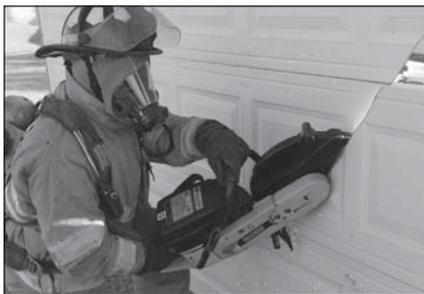
4. Next to the same starting point, make a second diagonal cut to the left, down to the bottom of the door. Fold the door down to form a large triangle.
