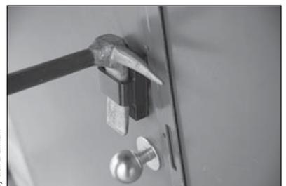
1. Size up the door and lock area, checking for any safety hazards. Determine which type of lock is used, whether it is regular or heavy-duty construction, and whether the lock cylinder has a case-hardened collar, which may hamper proper cutting. Place the K tool over the face of the lock cylinder, noting the location of the keyway.
