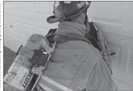
1. Before cutting, check for any safety hazards during the size-up of the garage door. Select the appropriate tool to make the cut. (The best choice is a power saw with a metal-cutting blade.) Wearing full protective gear and eye protection, start the saw, and ensure it is in proper working order.
